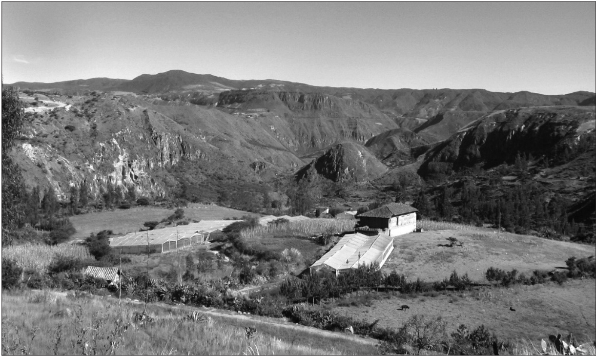
Buildings in the village are spread far apart from each other, making traditional sewer systems expensive and impractical.
